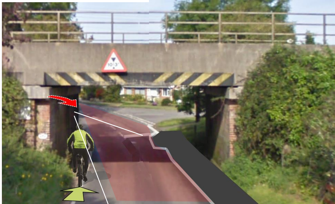
figure 7: Concerns expressed at earlier Committee meeting include – Will there be a blind spot under bridge where oncoming traffic [eastbound] will not see a cyclist [westbound]? [illustrative image – not to scale]
