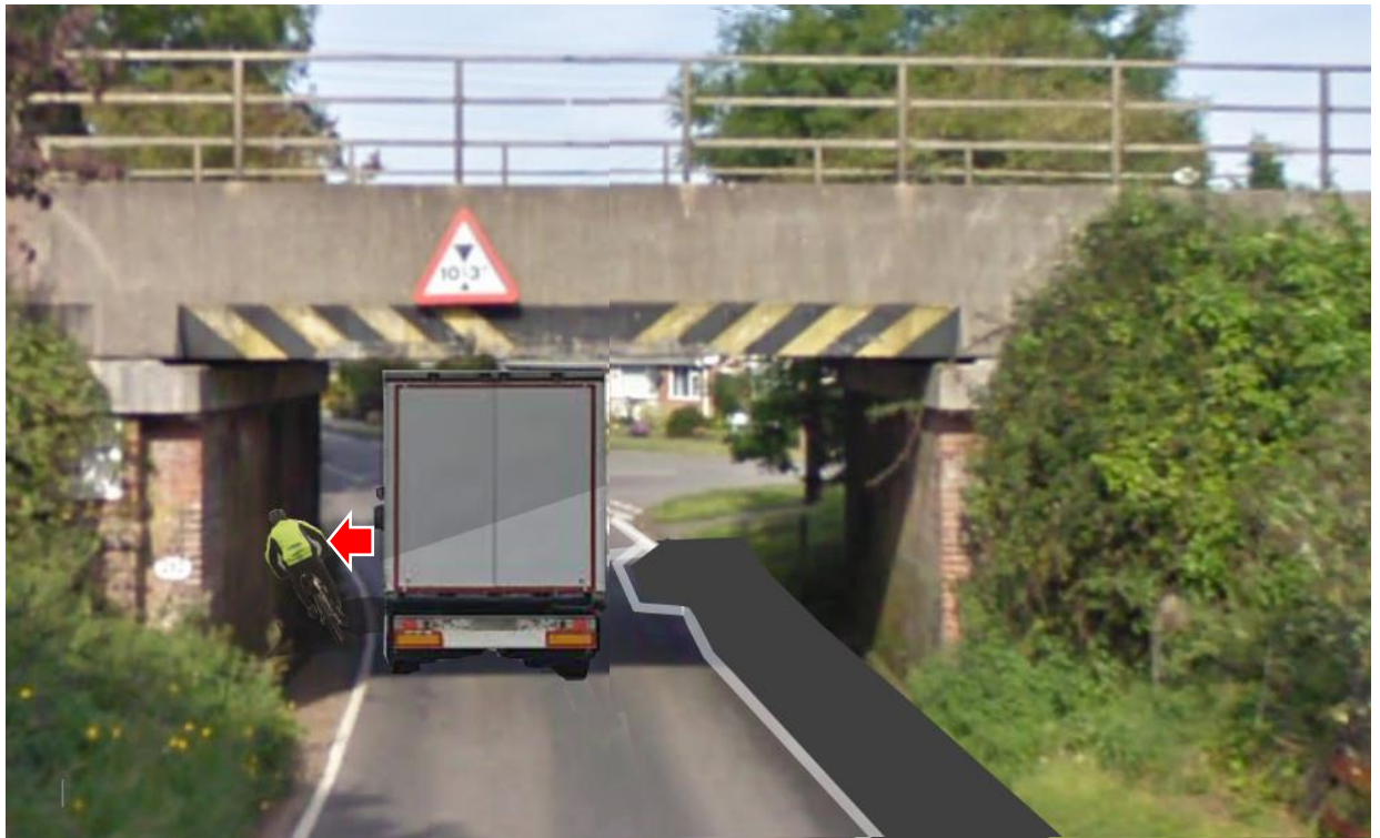
figure 8: Concerns expressed at earlier Committee meeting include – Will the proposed road narrowing expose westbound cyclists to the risk of being pushed up against the bridge abutment by passing/overtaking vehicles? [illustrative image not to scale]
